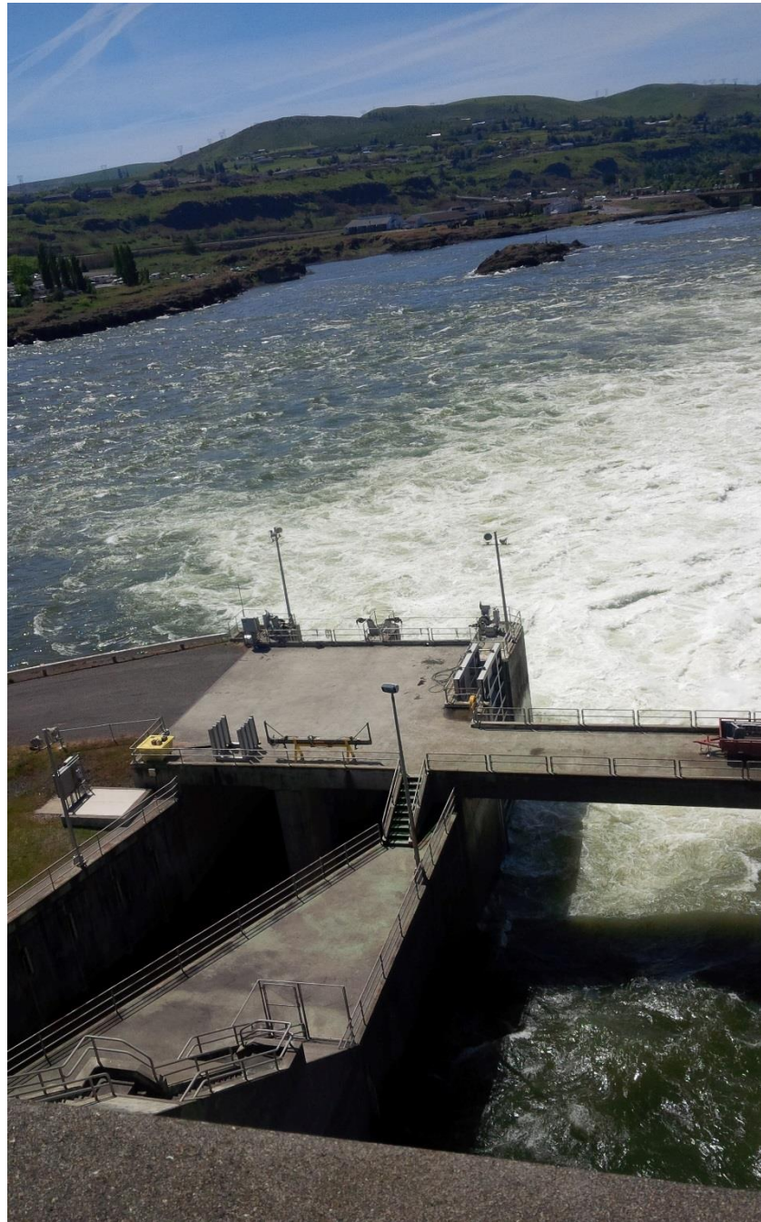
Spill turbulence near south entrance. Still very passable.
